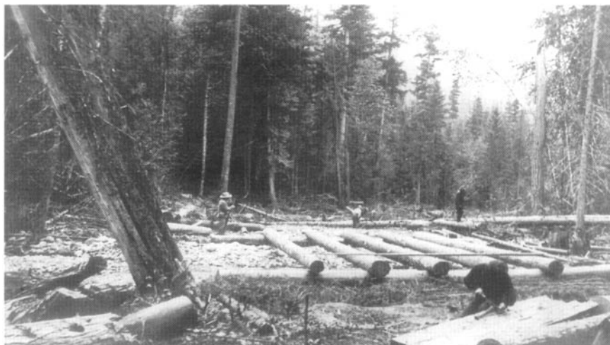
Road work, Mara Lake
