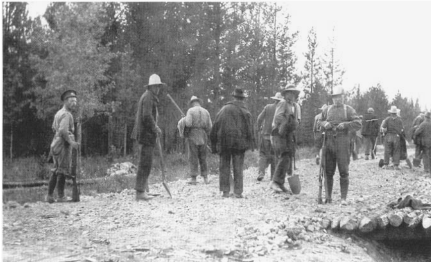
Work on Banff–Lake Louise Road, Castle Mountain
