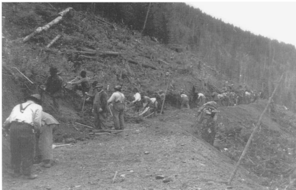
Road excavation, Monashee
