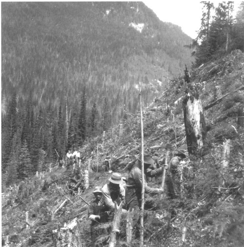
Grubbing on the Vernon-Edgewood Road, Monashee
